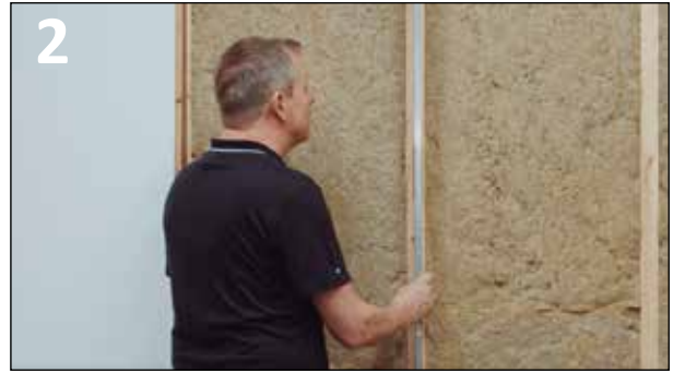
2 MAKE SURE WALL IS STRAIGHT AND LEVEL.
