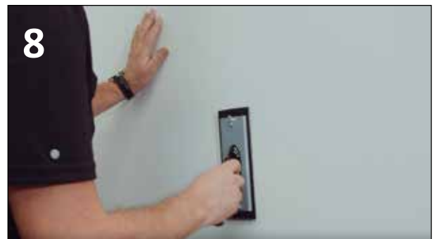
8 AFTER EACH BOARD IS FITTED, SAND LIGHTLY OVER JOINT BEFORE PAINTING OR WALL PAPERING.
