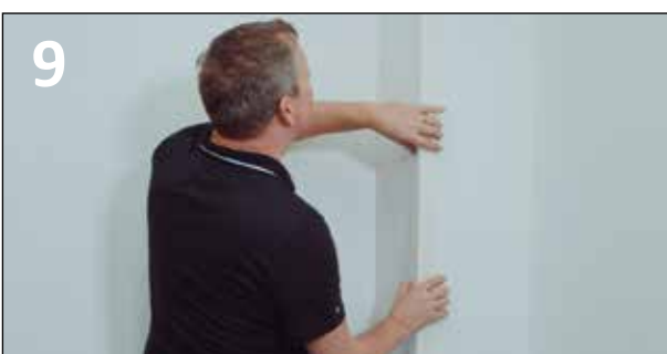
9 THE WALL CAN BE FITTED WITHOUT INTERNAL CORNER TRIM. FOR EXTERNAL CORNERS, OUR FLEXILIST CAN BE USED.
