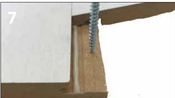
7 USE A 1MM STRING OF WOOD GLUE ALONG THE JOINT PROFILE. EACH PANEL MUST BE COMPLETELY FIXED TOP, BOTTOM AND SIDES BEFORE NEXT PANEL IS MOUNTED.
