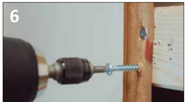
6 DOUBLE FIXING IN HORIZONTAL BATTENS.
